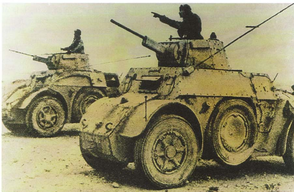
Two Italian Autoblinda AB 41 armoured cars on patrol in the desert. The main difference from the earlier AB 40 was the 20mm gun and coaxially mounted machine-gun in the turret in place of twin 8mm machine-guns. It was the most widely used Italian armoured car of the war. (Author's Collection)
